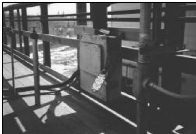
Figure 6 - Lock-out of cooling tower fan during accelerometer placement.
